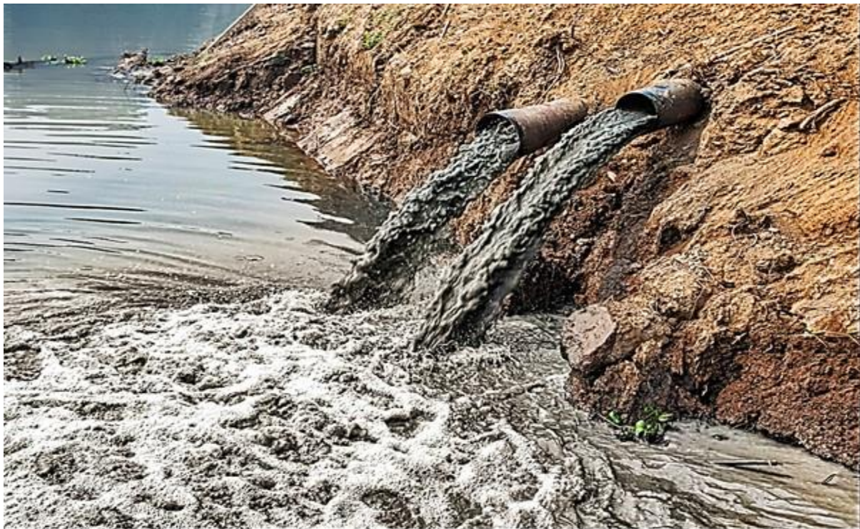
Fig. 10. Generic water discharge pipe with thanks to toa555 and Adobe Stock
