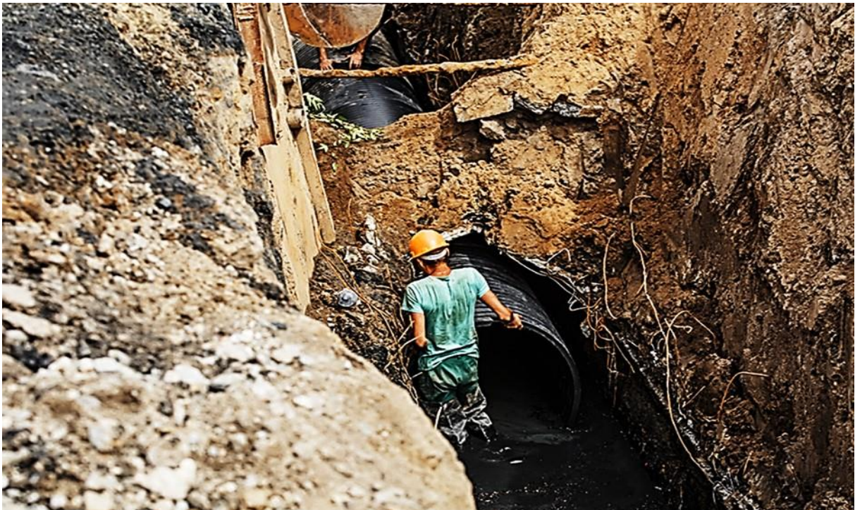
Fig. 15. Generic sewer relining with thanks to Oleksandr Bilyi and AdobeStock
