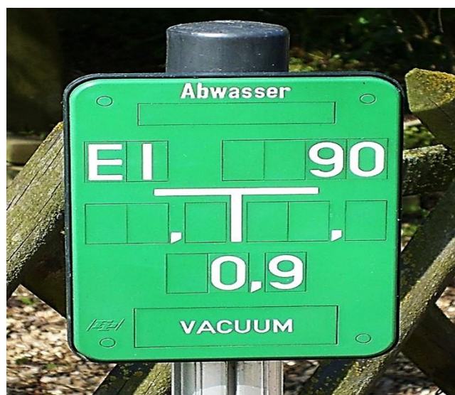
Fig. 28. Sign indicating a buried vacuum sewer in Germany, with thanks to C Lower and Wikipedia
