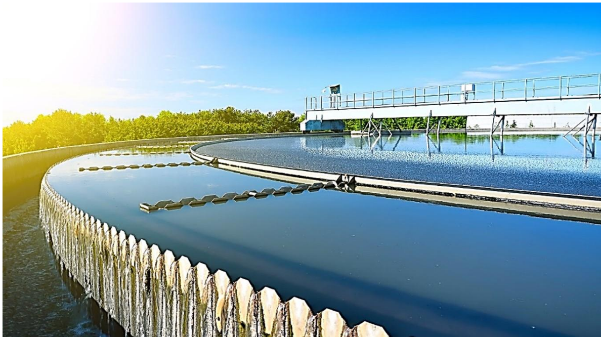
Fig. 24. Generic sewage treatment, with thanks to the Author and Adobe Photo Stock.
