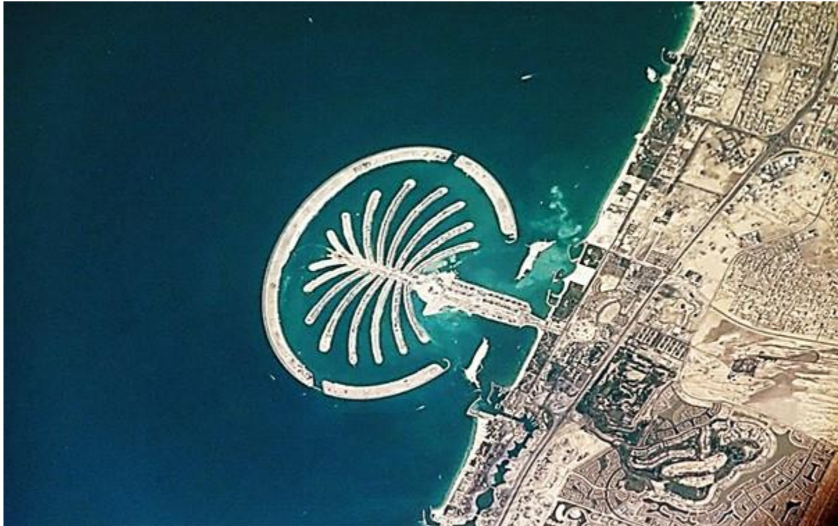
Fig. 31. Palm Island in Dubai, United Arab Emirates, is a vacuum WC project by Roevac. It features 2,300 villas, approximately 40 km of vacuum sewer lines, 1,050 collection chambers, and one central vacuum station. On completion in 2008, it was the world’s largest vacuum sewage installation (Mohr, 2016), thanks to NASA and Wikipedia.
