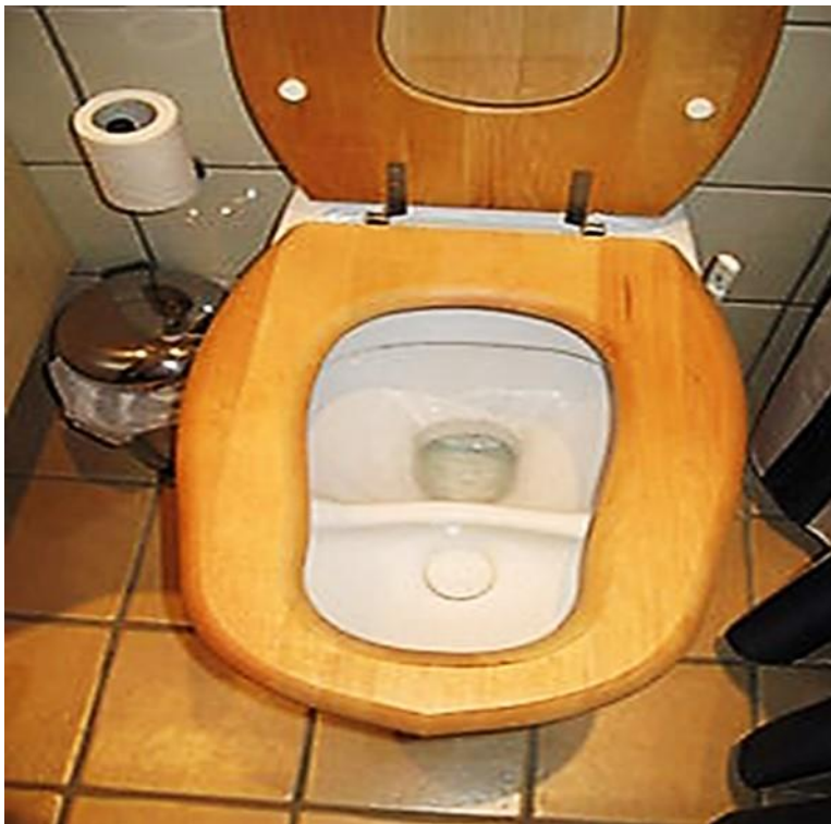
Fig. 32. Urine diverting toilet in Sweden with many thanks to the author EvM-Susana and Wikipedia
