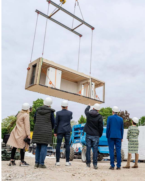
Figure 4: Site visit to the construction site of Kappesgärten primary school – district administrator Christian Engelhardt, the school management, the head of the municipal enterprise for schools and building management, with the project lead and the architect.
