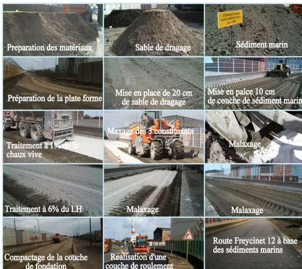
Figure 24. Stages of realisation of the experimental work based on harbour sediments
