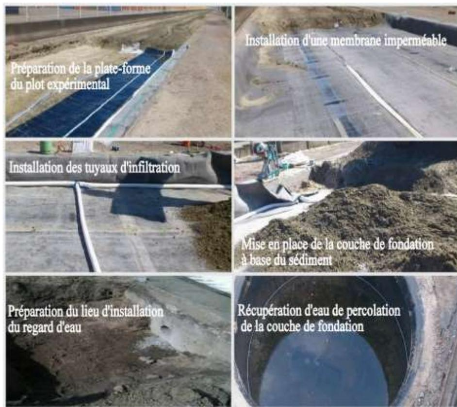
Figure 25. Stages of conducting instrumented experimental work
