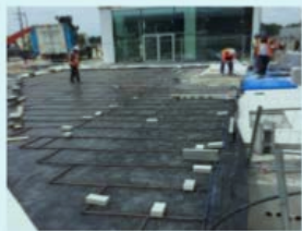
Installation of the injection network and evaporative pavements
