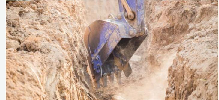
Excavation materials (most commonly comprised of soil, stone and gravel) produced in the construction activities can present a potentially large source of raw materials. These residual flows can be remanufactured into bricks to be used again in new construction.
